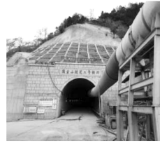
图2 洞口概况 Fig.2 Survey of the tunnel entrance
